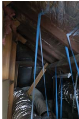
Figure 85.0, Roof space as accessed from attic showing Air Con ducting, AW 2018
