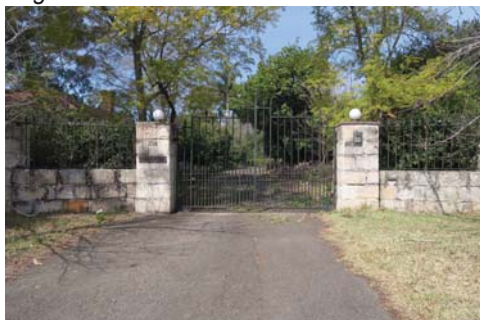
Figure 105.0, Entrance to Wood Martin, 104 Livingstone Avenue.
