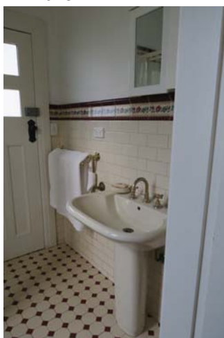
Figure 70.0, New laundry/bathroom fit-out, 1998, AW 2018
