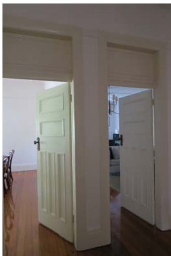
Figure 52.0, Original doors and fanlights, now painted, AW 2018
